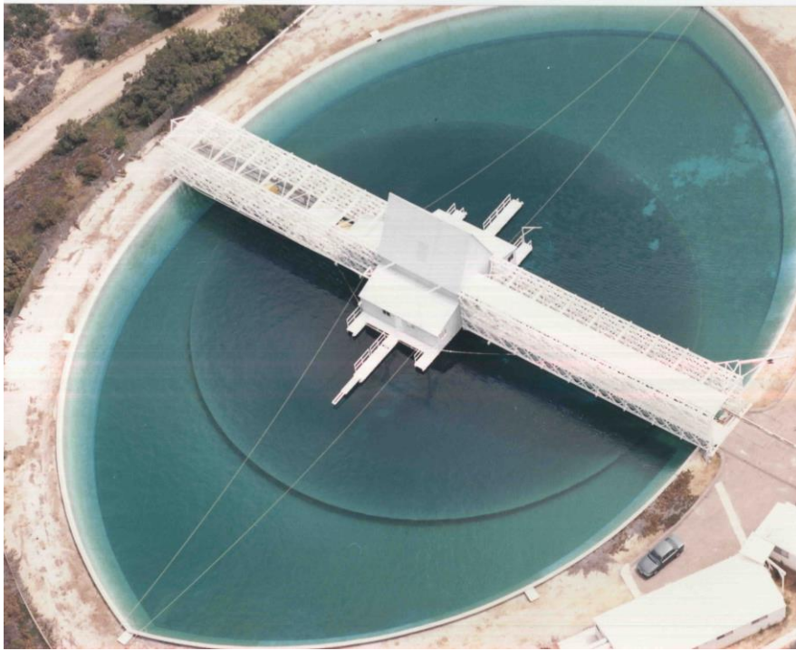
Figure 1: Aerial photo of facility. The bridge structure has no piers or supports in the pond.
